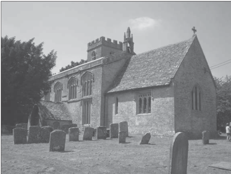
Idbury parish church from the south-east, showing the 12th century chancel and nave, 14th century porch, bellcote and tower, and 15th century clerestory.
